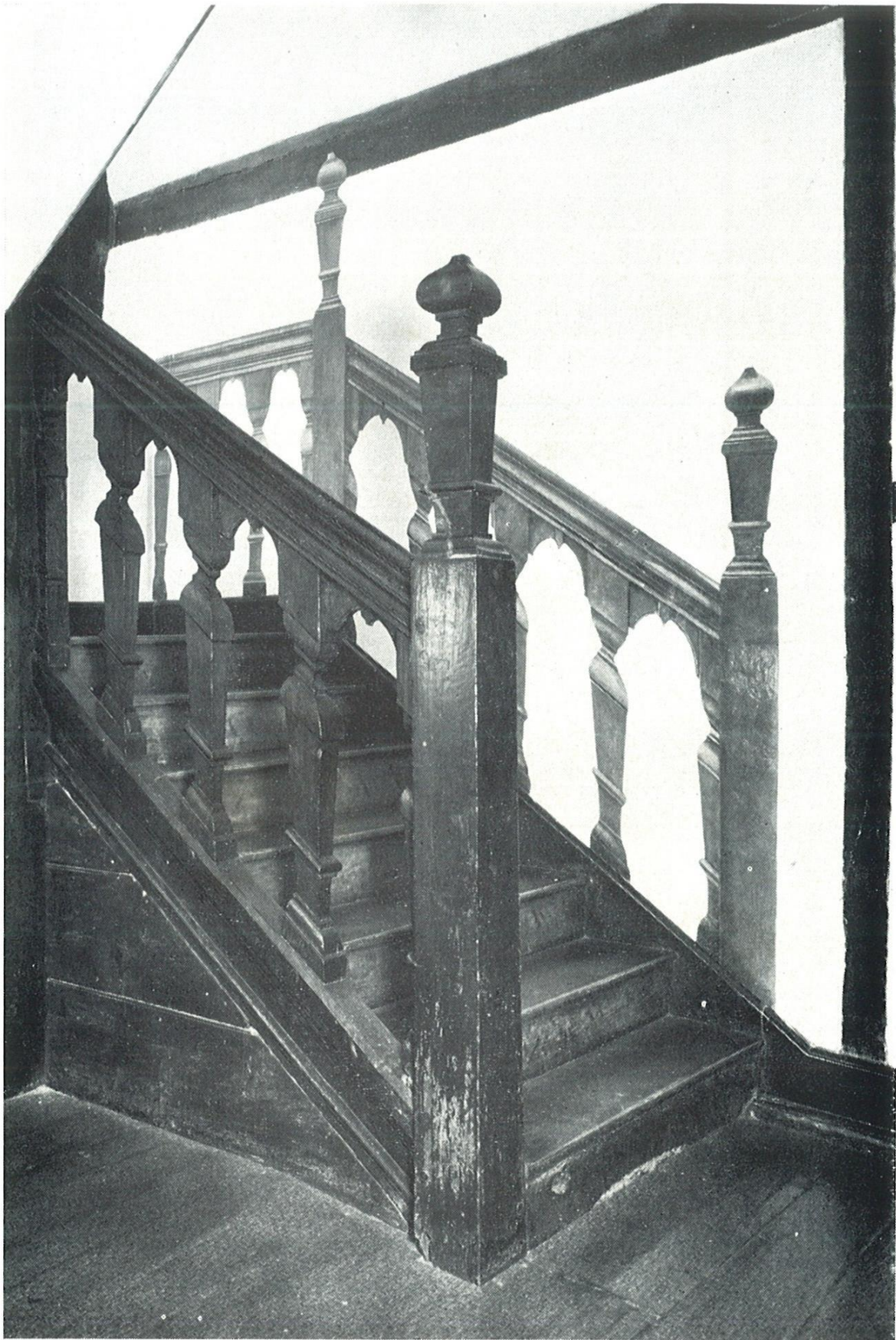
THE BACK STAIRCASE, SHOWING PAINTED BALUSTRADE
